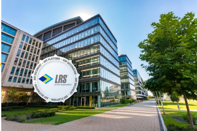
Apps and servers in central Data Centers
